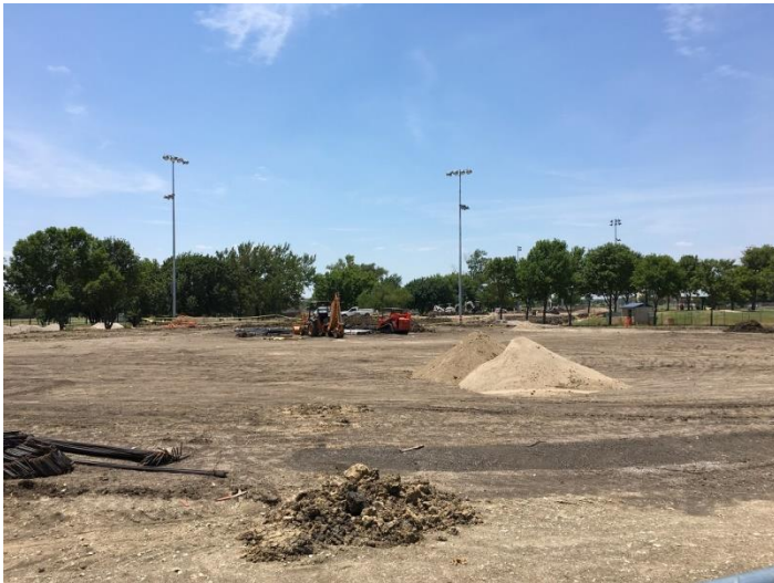
New Softball Field
